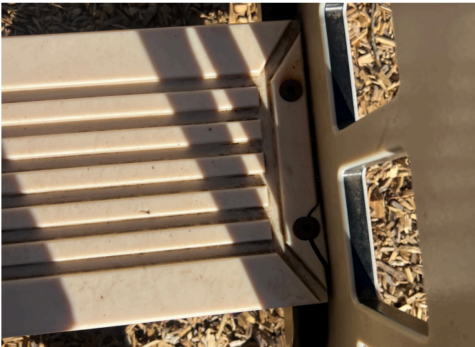
Above: non-compliant structures: playground safety codes from Consumer Product Safety Commission (CPSC) and American Society for Testing and Materials (ASTM) require the height of the slide exit region should be no more than 7" for preschoolers and no more than 11" for kids aged 5-12 to ensure safe transitions from the slide to the ground.
