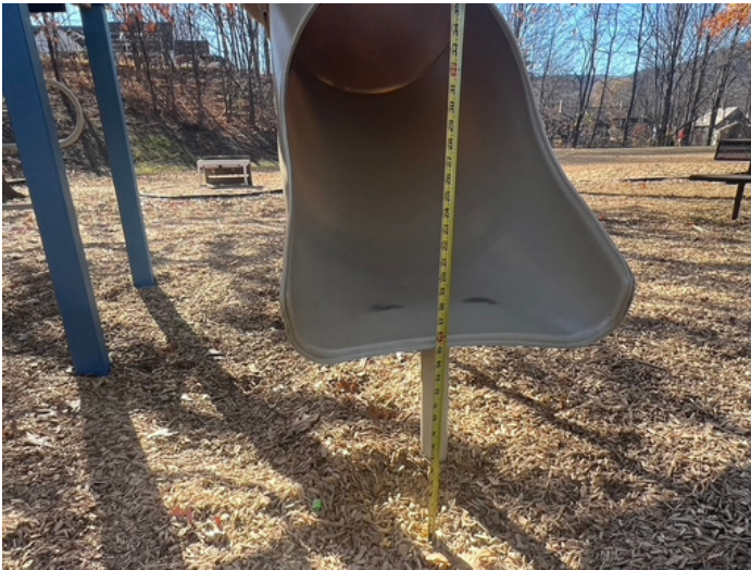
Above: non-compliant structures: playground safety codes from Consumer Product Safety Commission (CPSC) and American Society for Testing and Materials (ASTM) require the height of the slide exit region should be no more than 7" for preschoolers and no more than 11" for kids aged 5-12 to ensure safe transitions from the slide to the ground.
